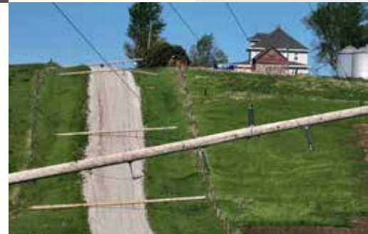
▶ A domino of downed poles line a gravel road.
